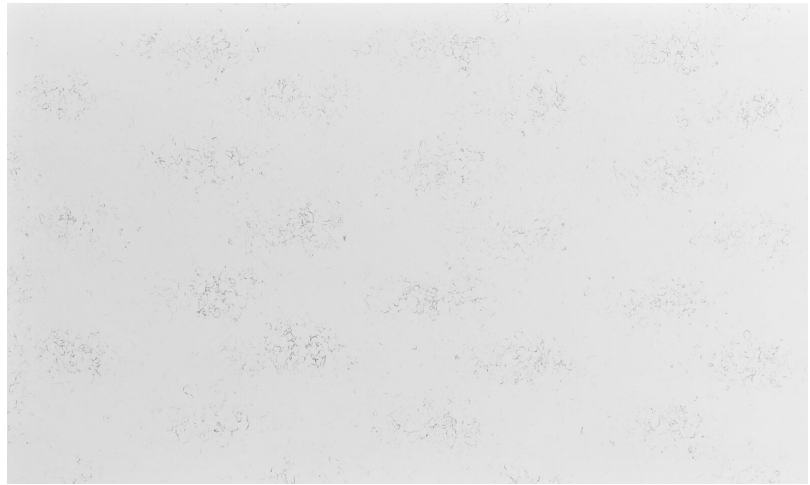
FULL SLAB VIEW
